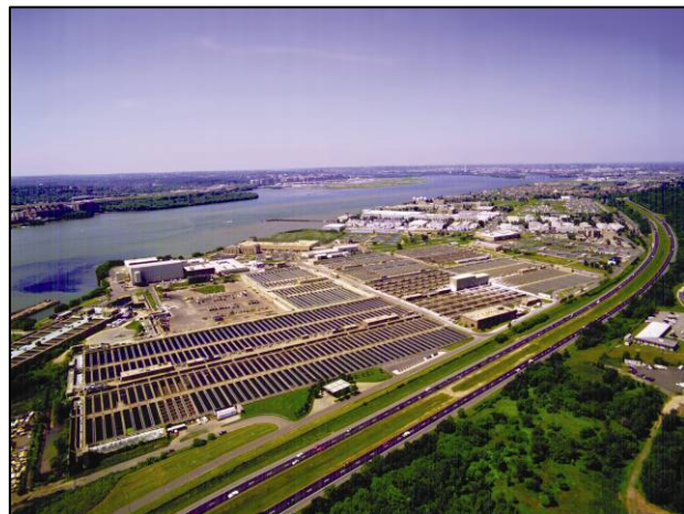
Aerial photo of Blue Plains Waste Treatment Plant
