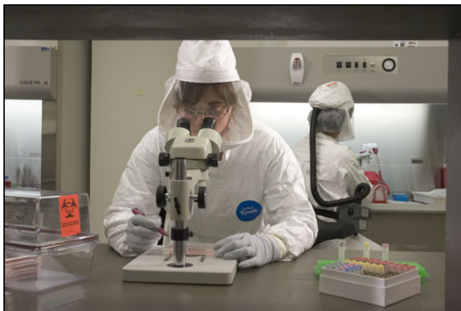
The Department of Health laboratory is in need of comprehensive upgrade to meet government standards for health and safety, particularly for the ventilation and operation of its Bio-Safety Level 3 tuberculosis laboratory.
