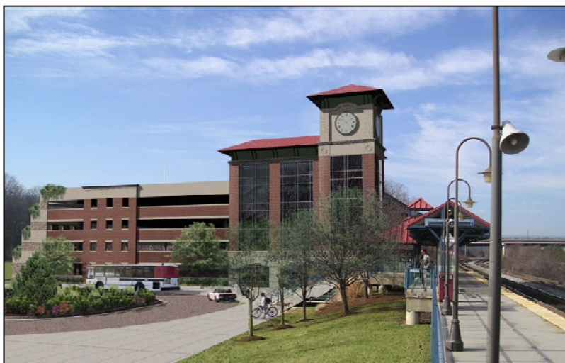
Burke Virginia Railway Express (VRE) Station.
