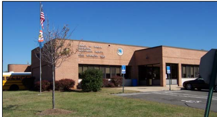
Picture of existing Newington facility
