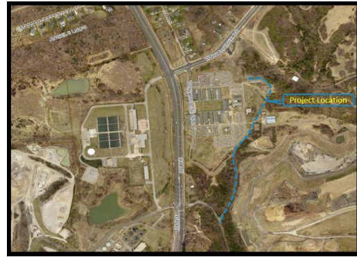
Workhouse Arts Foundation Cross County Trail Connection reaches substantial completion.
