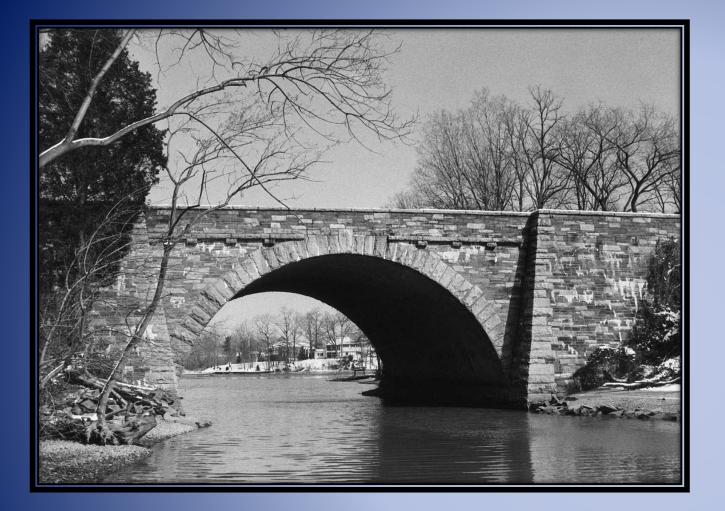
The Mount Vernon Memorial Highway is significant as the first parkway constructed and maintained by the U.S. Government and as the first such road with a commemorative function explicit in its name and alignment. Its distinctive stone-faced arch bridges, concrete slab base, beveled curbing, and landscape plantings mark its special quality.
