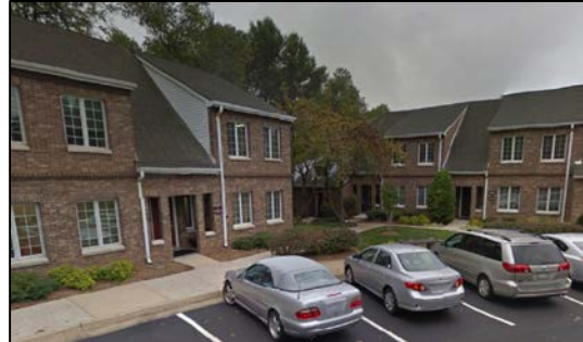
Office units along Bowman Green Drive
