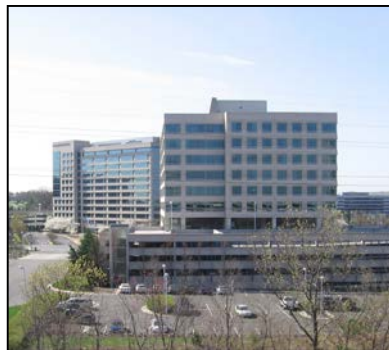
Two Discovery Square, a medium intensity office building and parking garage located in Reston Town Center.
