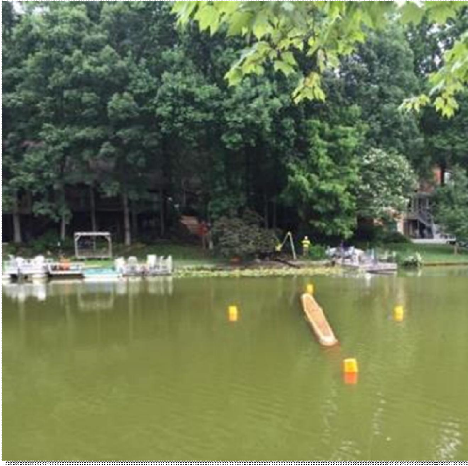
Lake Thoreau floated sewer line FY 2016
