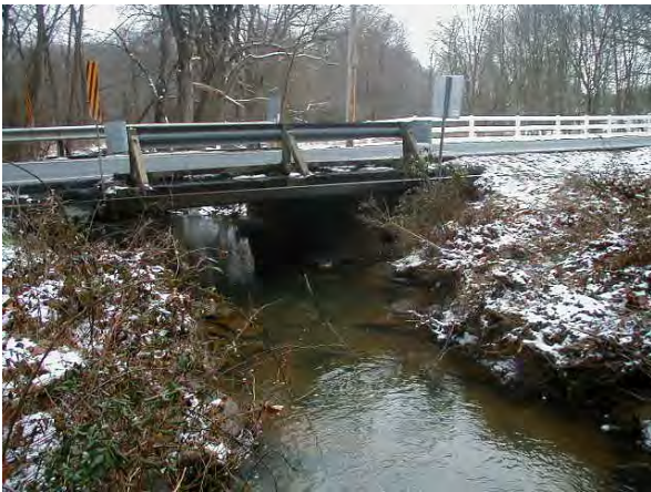
Photo 3.20 Piney Run Mainstem at Walker Road
