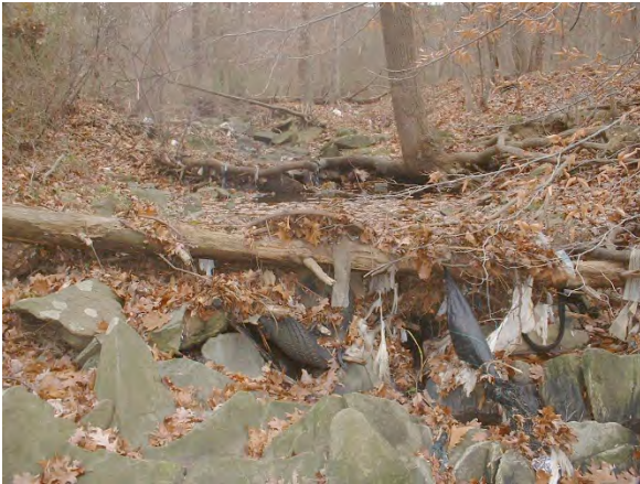
Photo 3.139 Stream blockage located upstream of the area shown in Photo 3.139 (DFDF043.T002).
