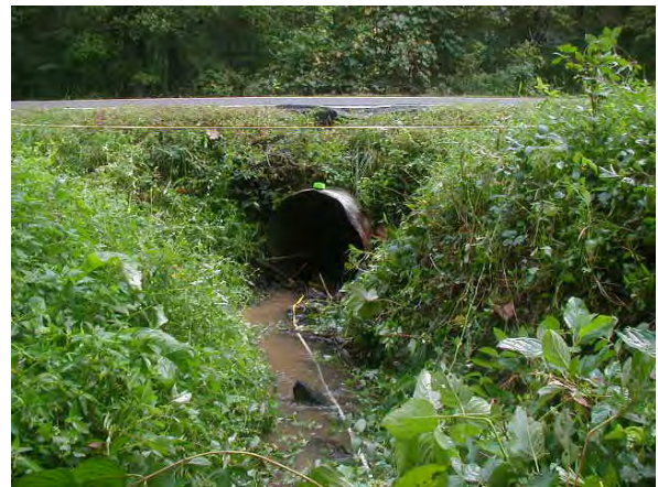
Photo 3.105 Little Difficult Run mainstem at Fox Mill Road North
