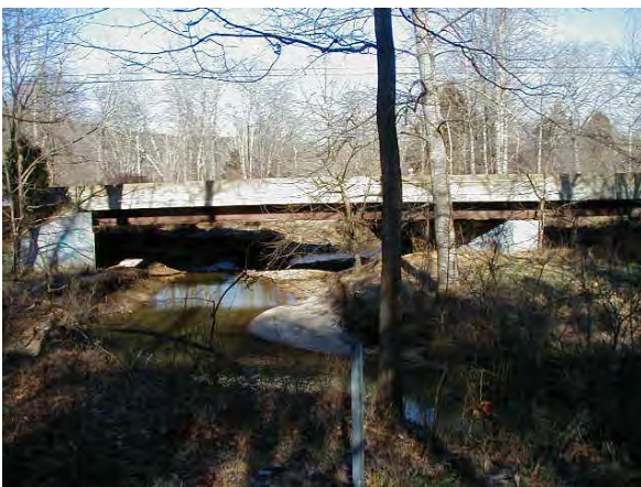
Photo 3.150 Difficult Run Mainstem at Vale Road
