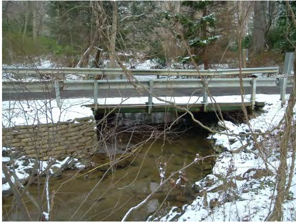
Photo 3.43 Culvert 76 on Rocky Run mainstem at Old Towlston Road
