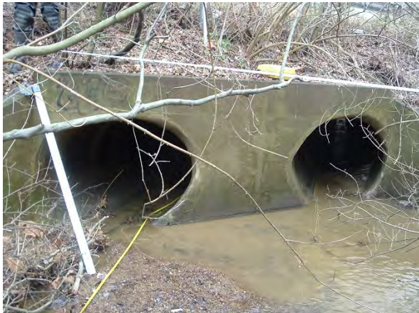
Photo 3.16 Piney Run Tributary at Riva Ridge Drive.
