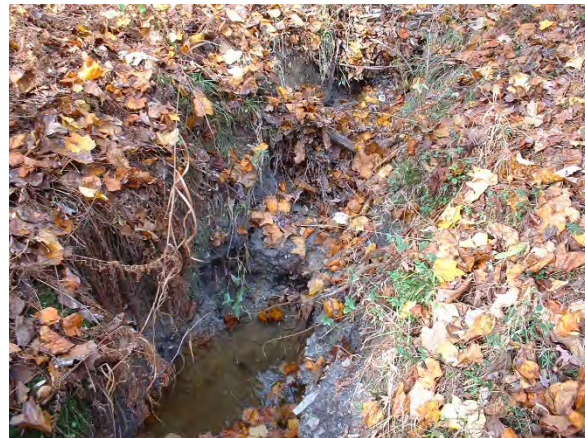
Photo 3.98 Headcut located northwest of Fox Mill District Park in the Fox Mill Woods subdivision. Directly east of the intersection of Steeplechase Drive and Aintree Lane (DFLD023.H001).
