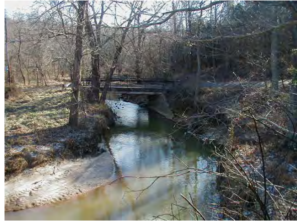
Photo 3.149 Difficult Run Mainstem at Vale Road
