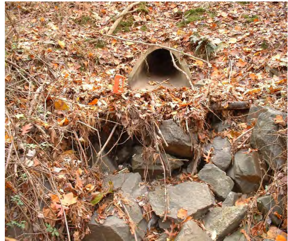
Photo 3.2 Erosion below stormwater pipe located at the end of Milburn Street (DFCH021.P001).
