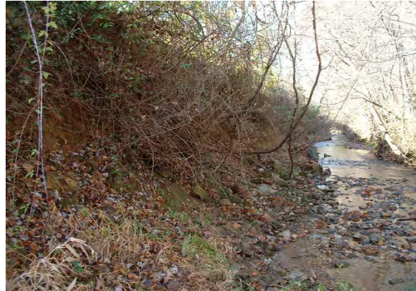
Photo 3.87 Streambank erosion just upstream from confluence with Difficult Run, west of Fosbak Drive (DFPB002.E001)
