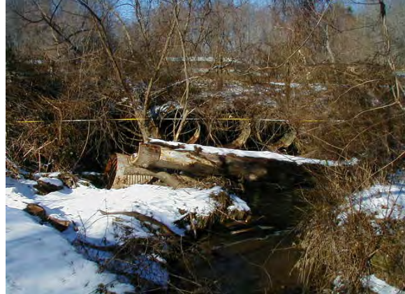
Photo 3.7 Unnamed Tributary at Sunnybrook Drive.
