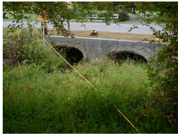
Photo 3.143 Difficult Run Tributary at Valley Road
