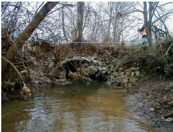
Photo 3.31 Lower Difficult Run Mainstem along Leesburg Pike
