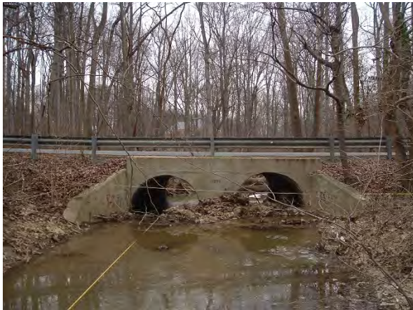
Photo 3.41 Culvert 74 at Brook Road on Rocky Run mainstem.
