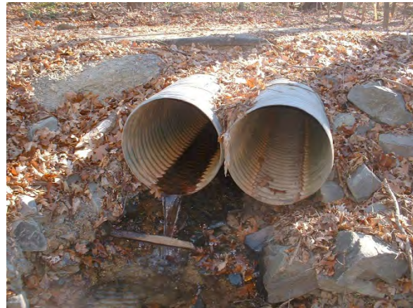
Photo 3.133 Pipe culvert between Lochinver Lane and Lakenheath Way.
