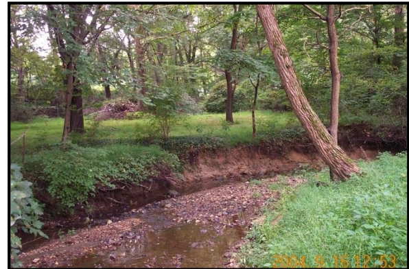
3-4' eroded bank with no buffer.
