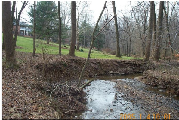
Eroded bank adjacent to mowed lawn.
