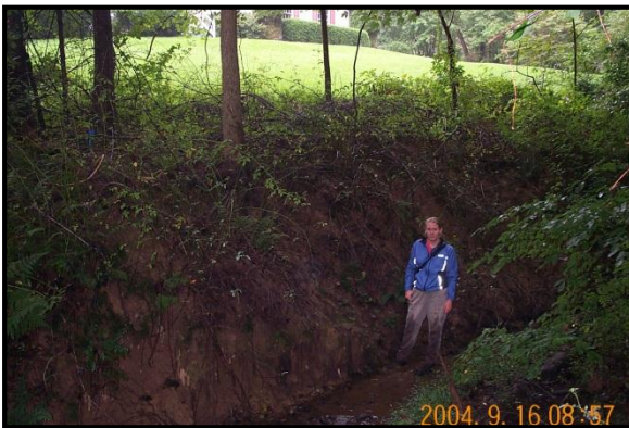
Eroded bank adjacent to Clifton Road.
