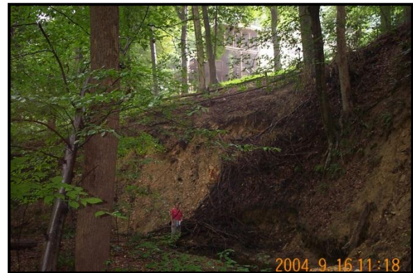
40' eroded bank near Havenner Road.
