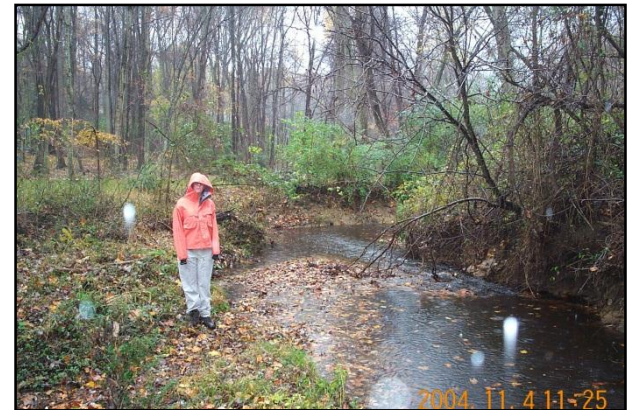
Stream erosion along outside bend.
