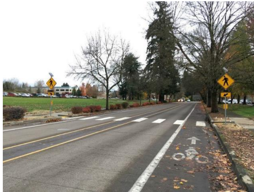
A mid-block crosswalk is a crossing that is located between two intersections
