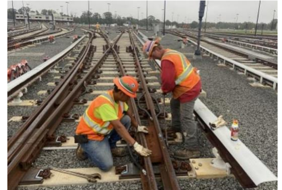
Finalizing Switch Alignment
