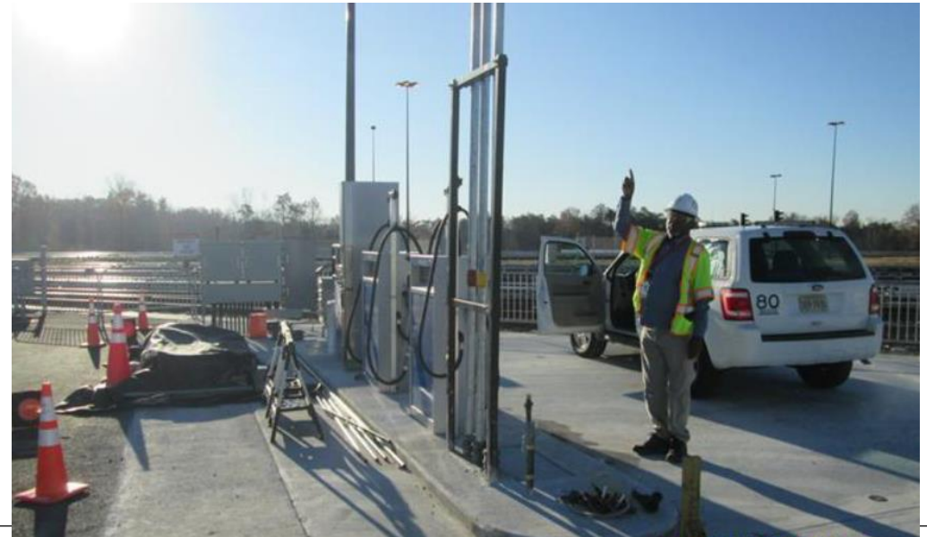
Inspecting Fuel Dispensing Point
